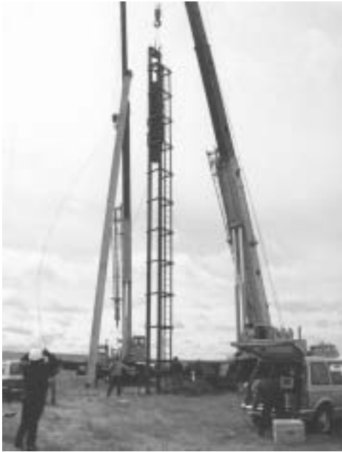
Fig. 8.2—View of installation of CFRP test pile (Iyer 1995).
