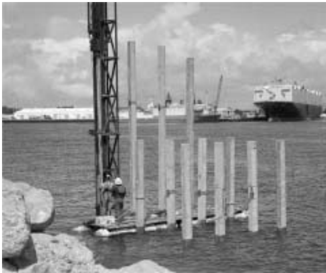
Fig. 8.3—Construction on CFRP prestressed piles supporting pier.
