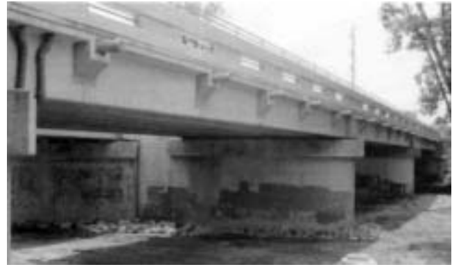
Fig. 1.5—Completed Bridge Street Bridge (Grace et al. 2002).
