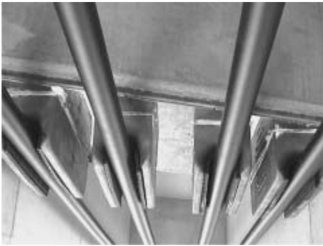
Fig. 7.1—Saddles used on the Bridge Street Bridge (Grace et al. 2002).
