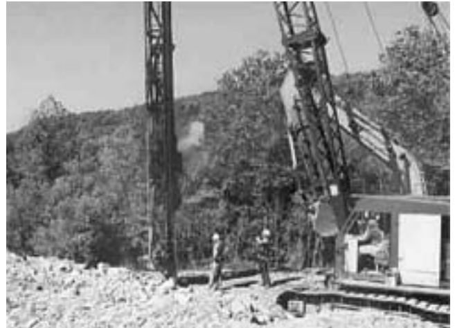
Fig. 8.6—View of installation of hybrid CFRP/steel (Schiebel and Nanni 2000).
